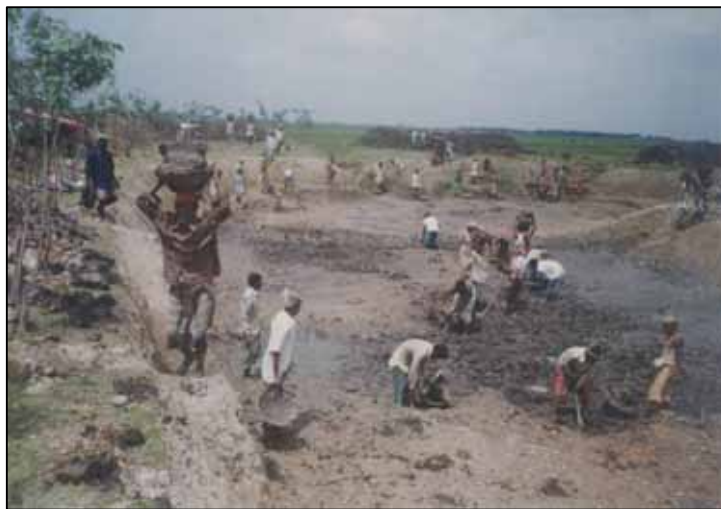
About 1.8 million person days of work was created through manual excavation of silted up wetlands
