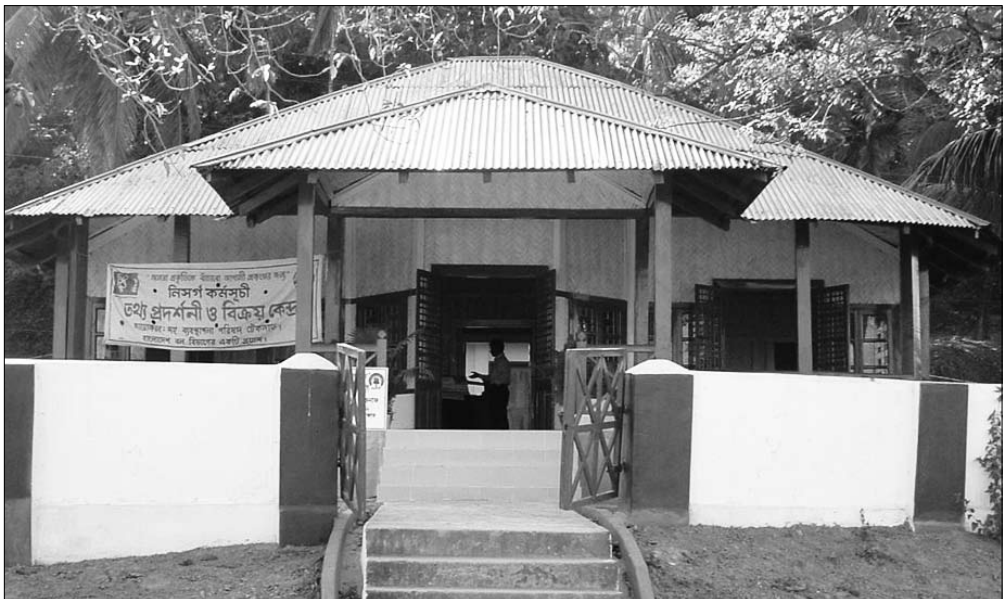
Forest Department staff bungalows like this one at Teknaf Wildlife Sanctuary were constructed in the 1920s. [Philip J. DeCosse]
