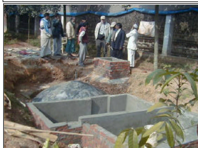
Constructing a biogas unit with FTF technical advice.
