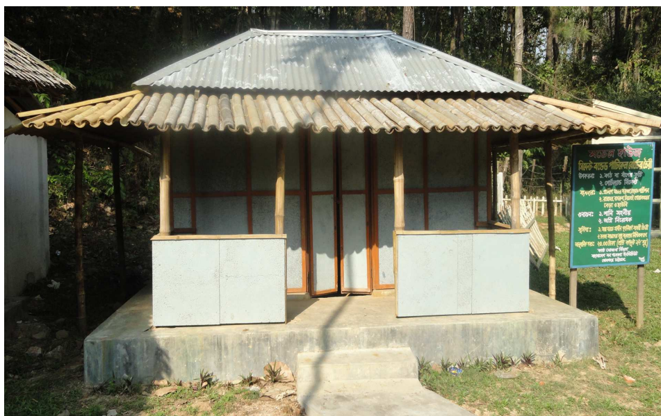
Figure 1. Model house-made of Cement bonded Particle Board
