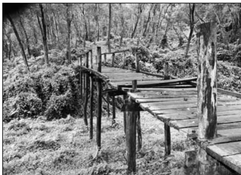
The old bridge which was built without following proper guidelines was unstable and dangerous for visitors. [Quamrul Ahsan]
